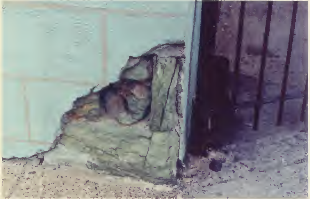
West Façade of Church Building (D)
